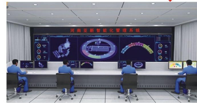
Monitor Room On Top of Kiln
