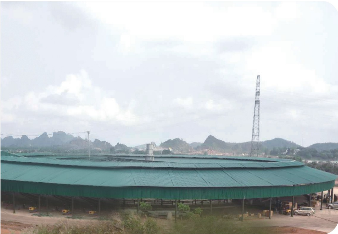
Project: Uzbekistan Rotary Kiln Location: Tashkent Kiln Section: 12.98m Kiln Capacity: 800000 bricks /day Materials: mountain earth, coal gangue
