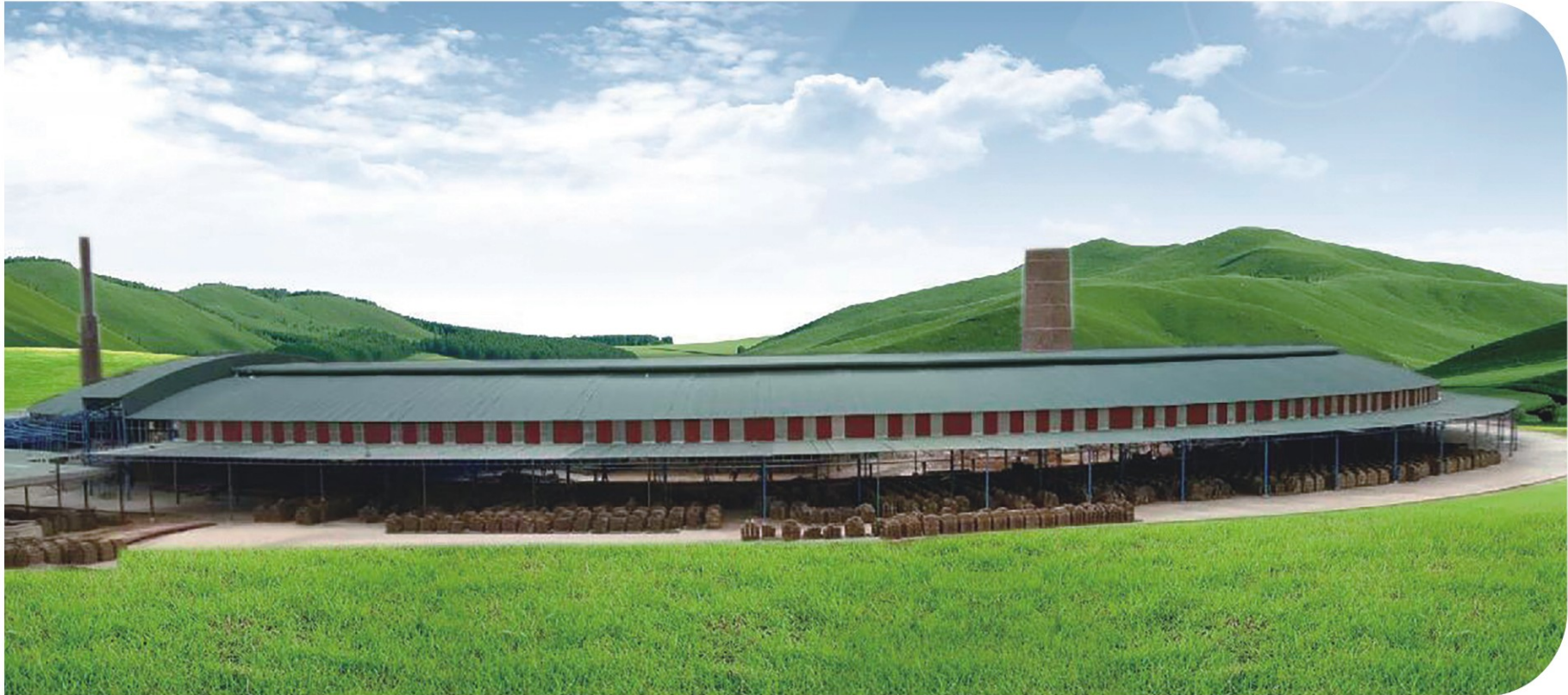
Project: Quang Binh, Brick Factory Location: Quang Binh, Vietnam Kiln Section: 11.8m Kiln Capacity: 400000-500000 bricks /day Materials: shale, river sludge, construction waste, industrial tailings
